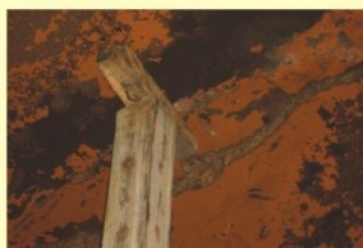
Ceiling Being Supported by Wooden Props
