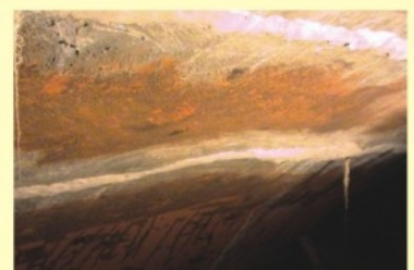
Final Structure after treatment
