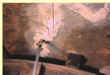
Grouting on process
