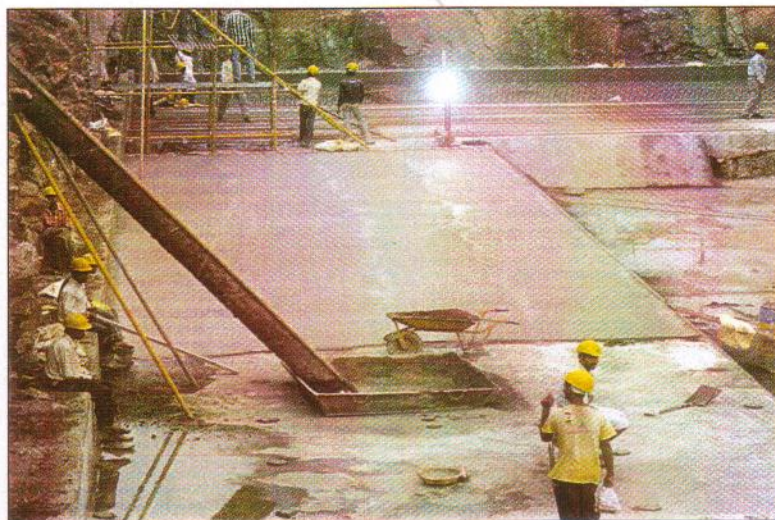
Waterproofing Work In Progress
